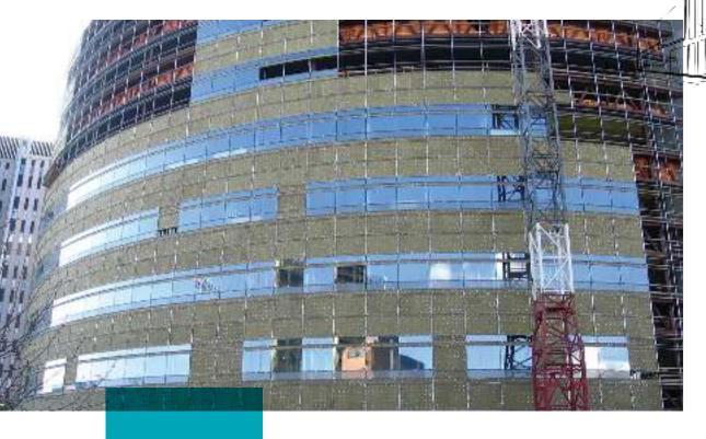
ROCKWOOL ROXUL SAFE™ is a lightweight, semi-rigid stone wool insulation that provides fire-stopping and acoustical properties. It is designed to fill perimeter gaps between concrete floor slabs and exterior wall systems, between firewalls and ceiling slabs, and around conduit pipes and duct openings through walls and floor slabs.
